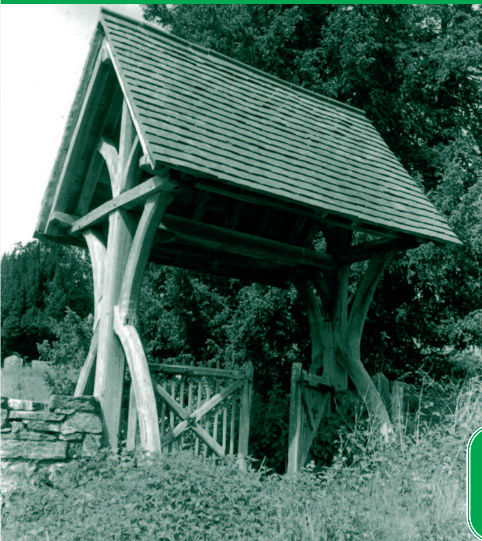
Lychgate at the church of St James, Tedstone Delamere, Herefordshire.
